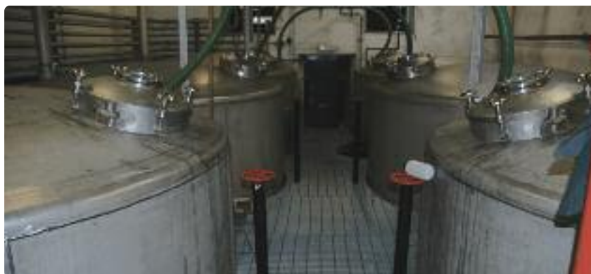
Left: Wash and spirit stills. The inset shows the 'steam kettles' in wash still.
